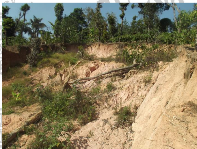
(b) Earth slide occurred in cultivated land on moderate slope by water saturation in Megatalu village
